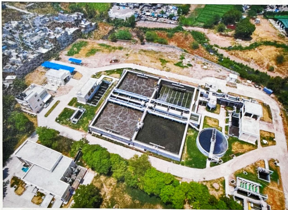
STP RAIPUR KALAN - I
